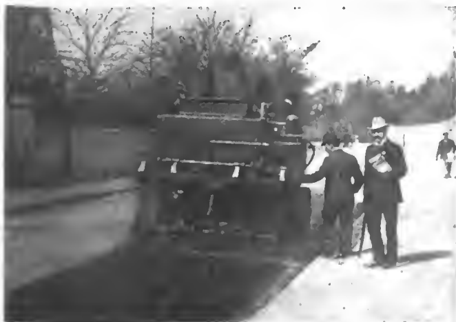
TARSPRA MACHINE, WHICH SPREADS THE TAR UNDER PRESSURE.
